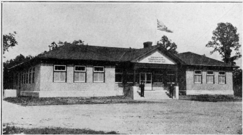
Windsor Park Golf Club House destroyed by fire. This photo was taken just after the building was erected and does not do it justice. Lawns, shrubbery and flowers in profusion had recently made a beauty spot of the surroundings.
