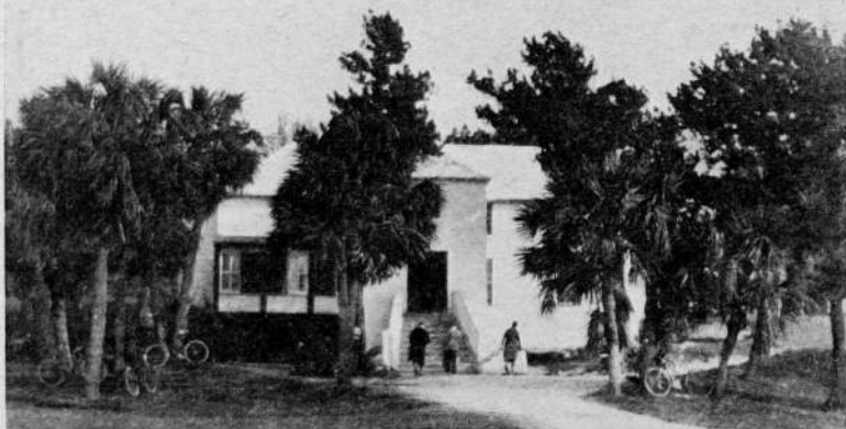
Garrison Golf Club House—One of the oldest houses in Bermuda.
