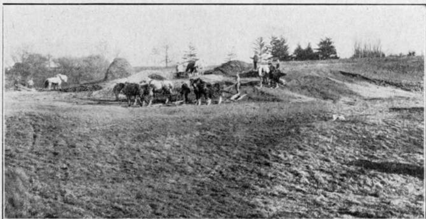
A construction gang at work on the eleventh green at the Royal York course.
