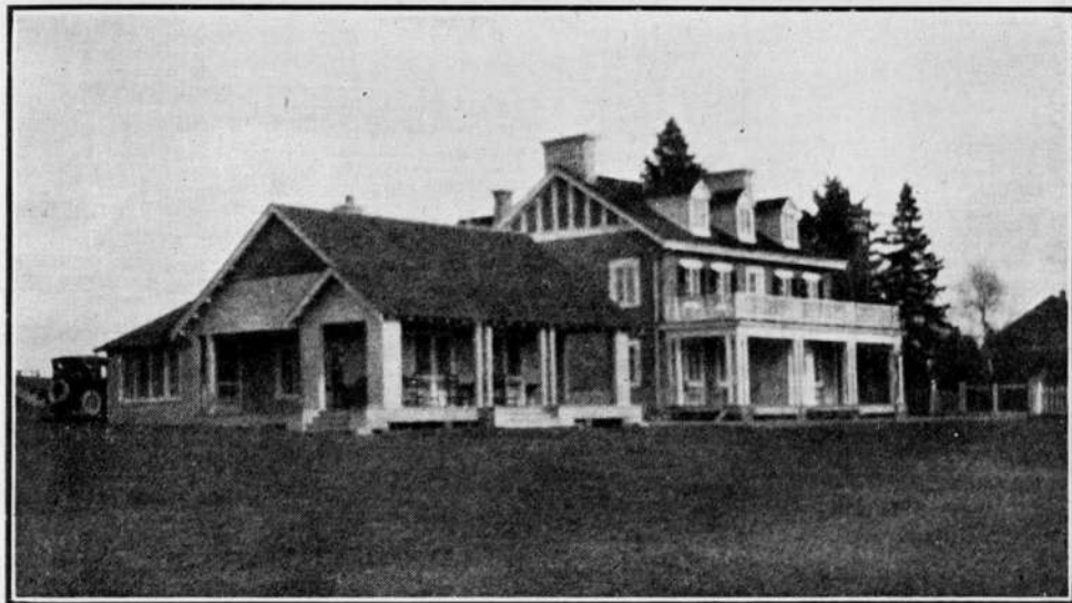
Quebec Golf Club House Destroyed by Fire. The Ladies' Building seen to the left of the Picture Was Fortunately Saved.
