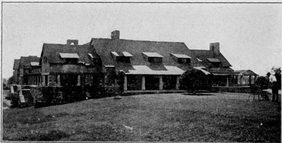
The dignified club house of the Beaconsfield Golf Club at Pointe Claire, Que., destroyed by fire this month. The loss is approximately $100,000.
