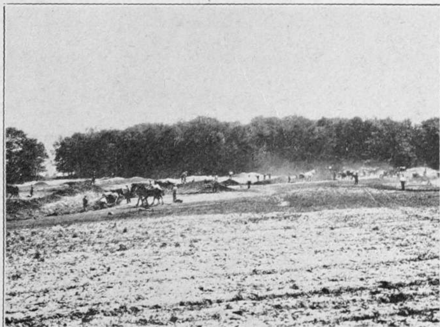
NEW GLEN MAWR COURSE, TORONTO—CONSTRUCTION WORK AT NINTH AND EIGHTEENTH GREENS
